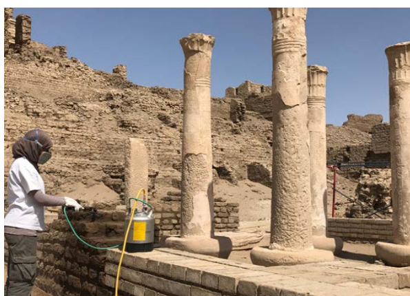
Figure 37: The conservator during the consolidation of old mud brick walls by ethyl silicates using the dispenser (a, b).
