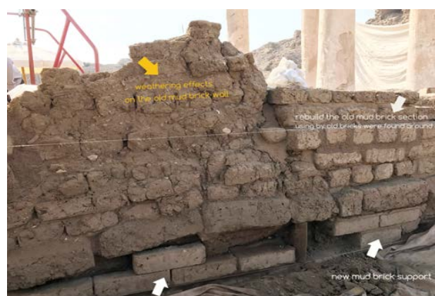
Figure 33: Shows the condition of the inclined wall in action to be restored & supported.
