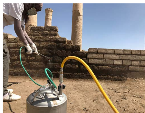
Figure 37: The conservator during the consolidation of old mud brick walls by ethyl silicates using the dispenser (a, b).
