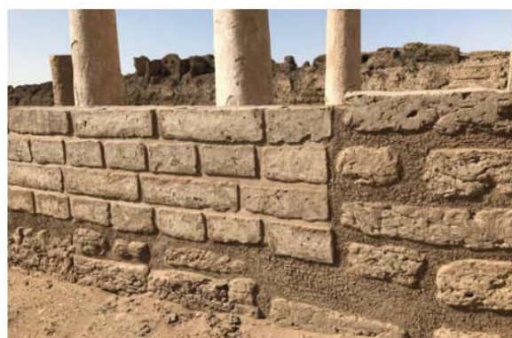
Figure 36: The conservators during the filling of gaps and joints using clay mortar for adobe wall (a, b), the wall after restoration; old parts and new section reconstructed using new mud brick, (c, d).
