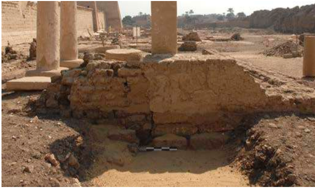
Figure 14: The state of conservation of the old mud brick foundation before the restoration works.
