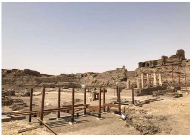
Figure 48: The construction of wooden bridge on archaeological features to protect it and to do way to reach the walkway to visit the butehamon house.
