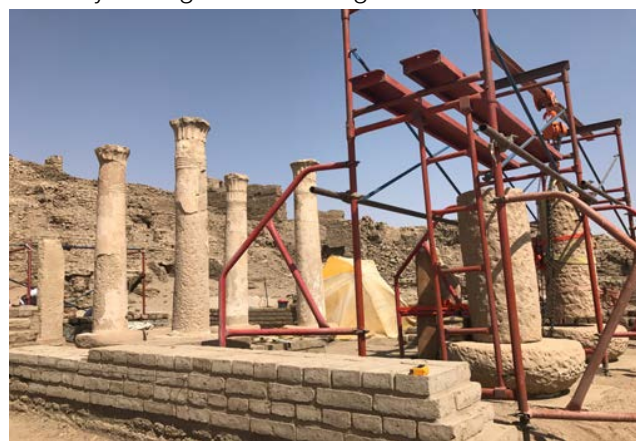
Figure 41: Shows the replacement of the two columns (with large parts missing) that were laid on the ground in final phase.
