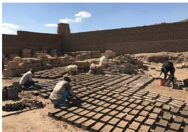
Figure 31: Workers add the mixture (clay & straw) to the mold for making adobe bricks.
