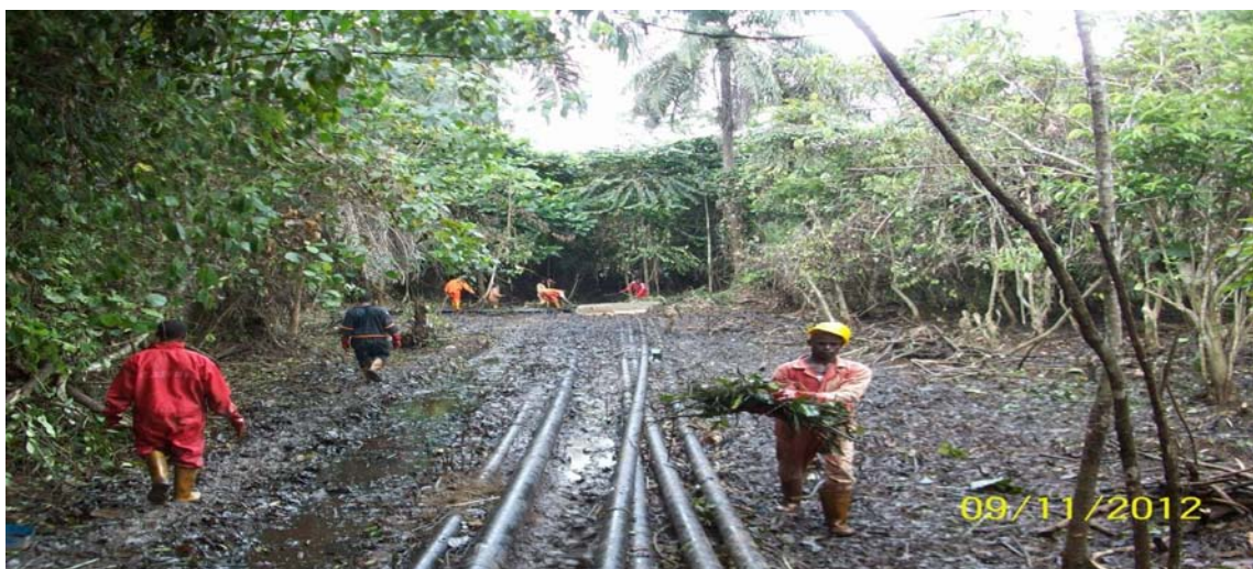
Figure 4: Right of Way Spill Clean up
