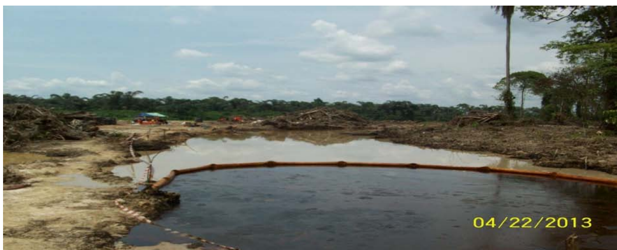
Figure 9: Oil Containment and Recovery in Progress
