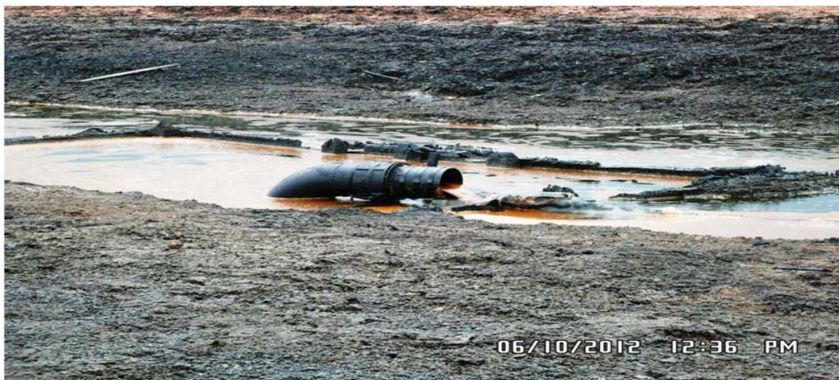
Figure 7: Inland Water Spill Due Cut Pipeline by Sabotage
