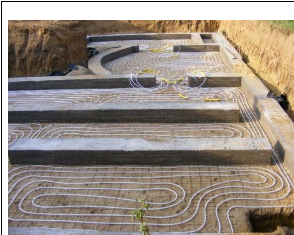
Figure 3a: Hydronic tubing before concrete pouring. Photo T. Barkanyi
