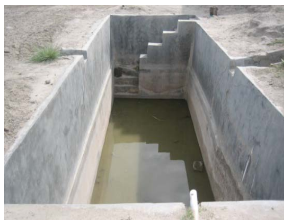
Figure 5 : Open storage water tank for collection of rain water
