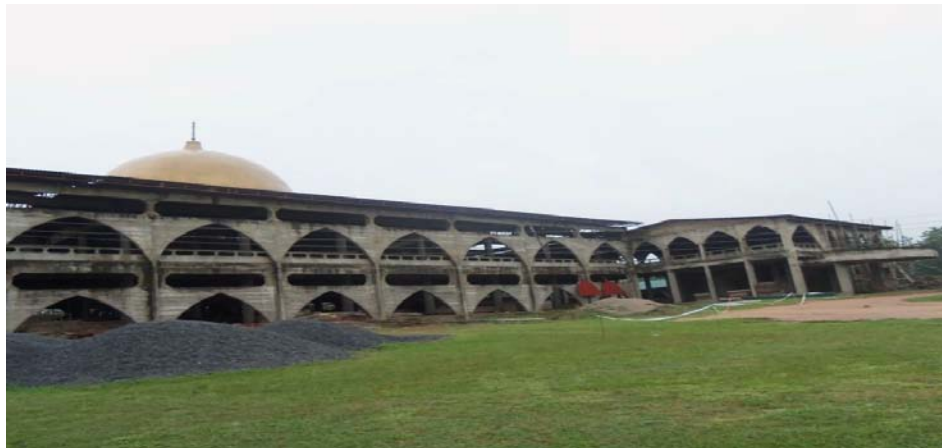
The new central Mosque under construction 3
