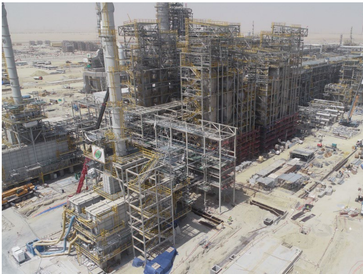
Fig. 11: Al Zour oil refinery project (ZOR) in the study area at Az Zour area southern Kuwait (Al Zour Refinery Project (ZOR) - Hydrocarbons Technology (hydrocarbons-technology.com)).
