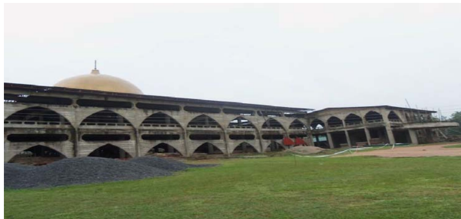
The new central Mosque under construction 3
