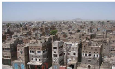
Figure 2: Panorama of Old Dhamar City and its Architecture [24]
