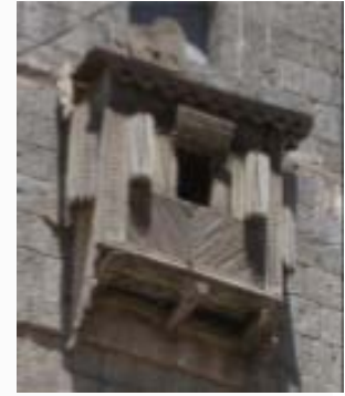
Figure 6: The Mashrabiya in the Façade [21]
